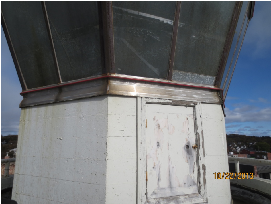
Photo No.5 Existing glass panels and access door
