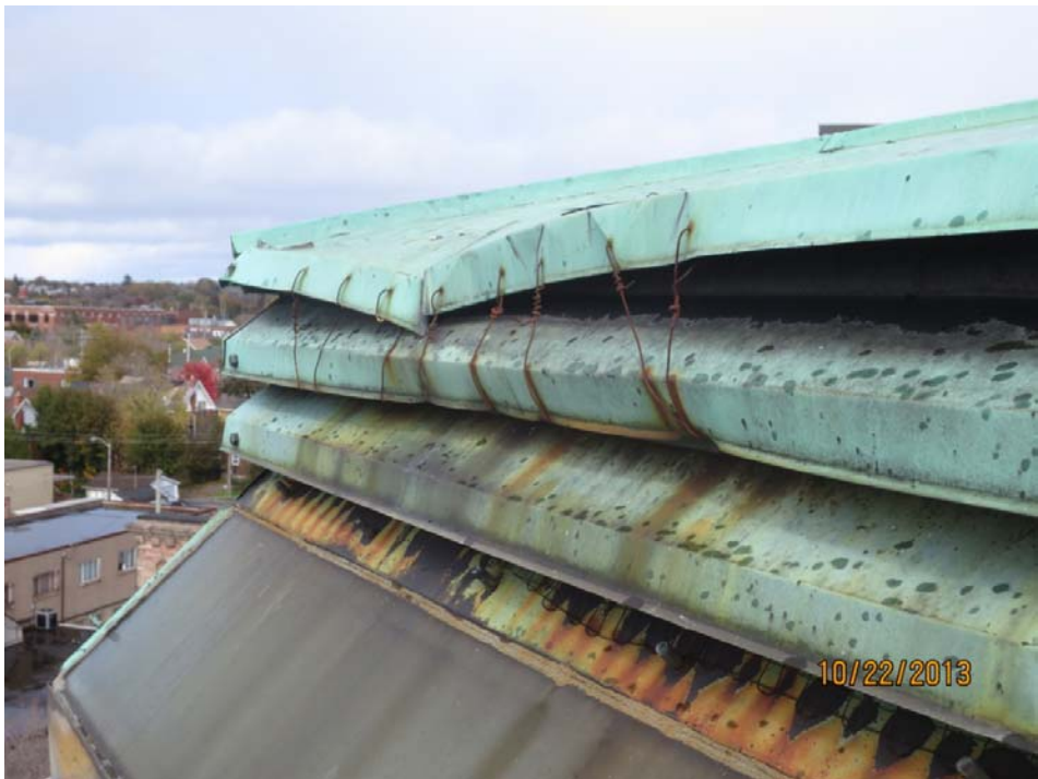
Photo No.6 Repaired copper roof cladding
